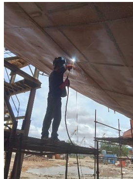
Figure 1. Overhead SMAW Welding Process
